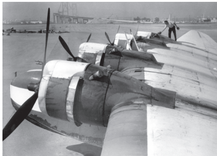
Dick Probert taking 881 out of mothballs at Reeves Field before the start of the summer tourist season. Note the Vincent Thomas Bridge under construction in the background. (Photo from Dick & Nancy Probert collection).
