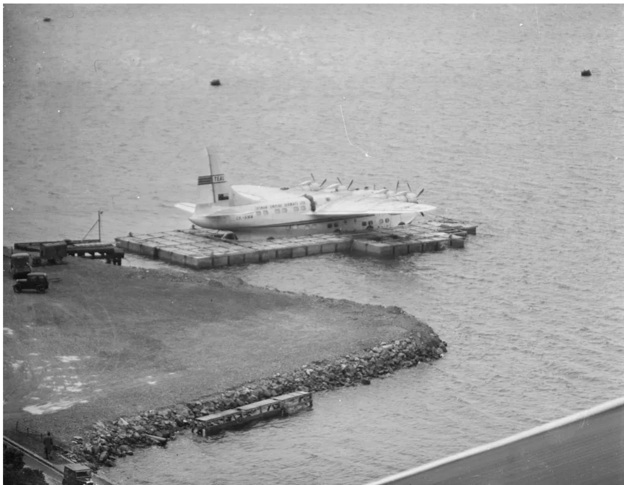
Another view of TEAL Solent ZK-AMM Ararangi undergoing repairs in the incomplete pontoon at Evans Bay.
