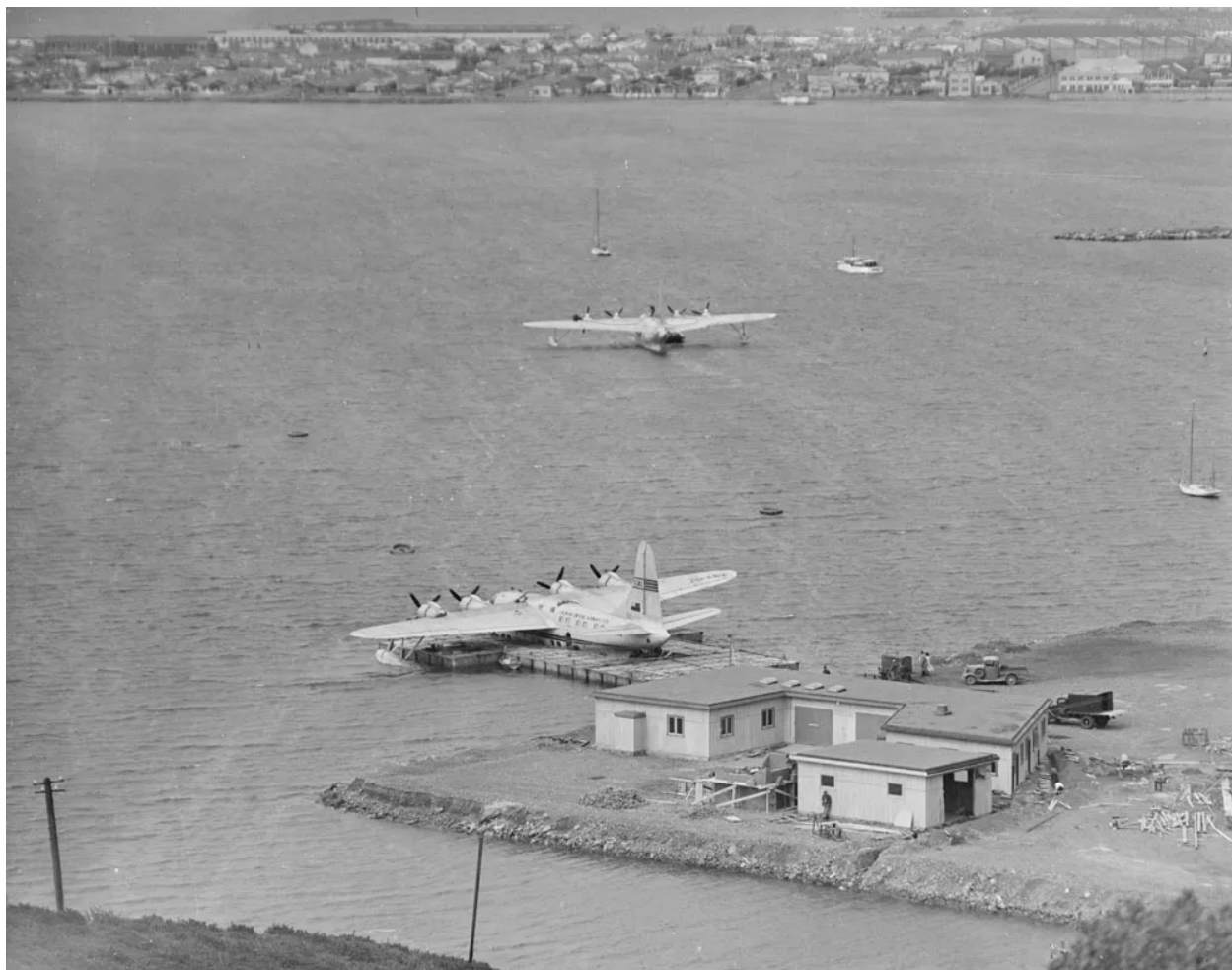
TEAL Solent ZK-AMM Ararangi undergoing repairs in the incomplete pontoon at Evans Bay on 19 October 1951. ZK-AMO Aranui can be seen moored to a buoy out in the bay.
