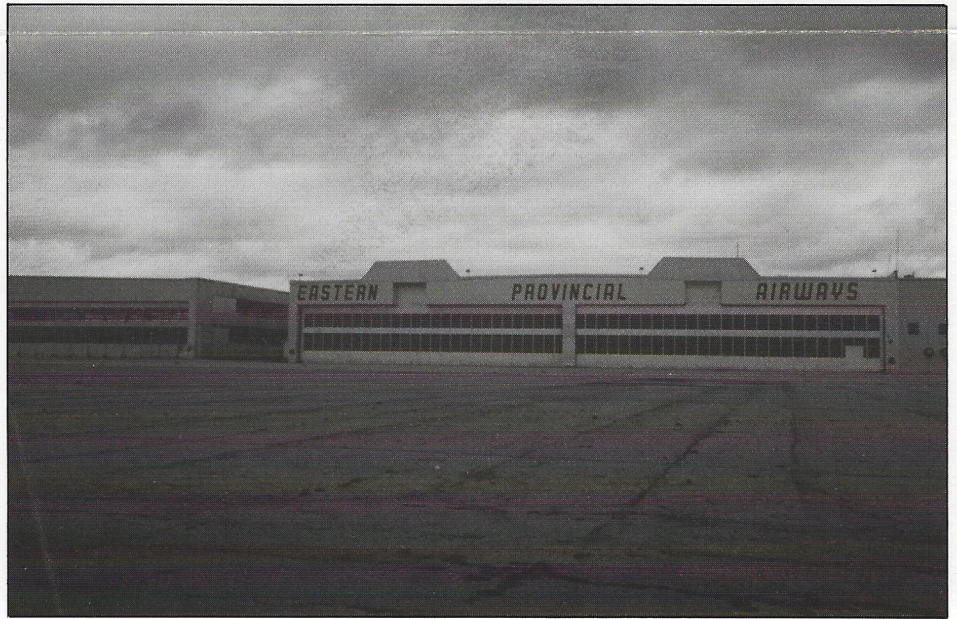
The future site of Hemmeter Aviation's full-service FBO and hangar, presently undergoing extensive renovation.
