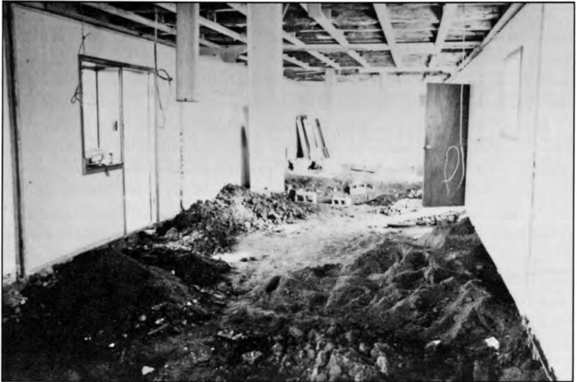
Figure 1.8 Interior of Building 14 after razing. Fill dirt is being added preparatory to pouring a concrete slab floor.
