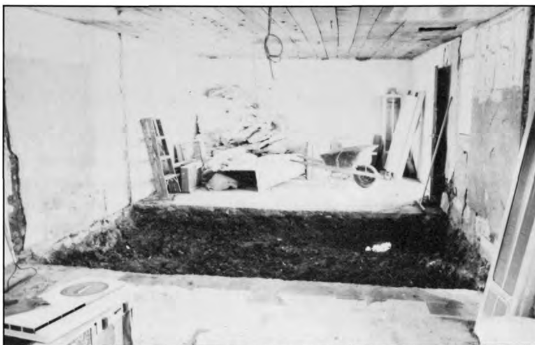
Figure 1.10 Interior of Building 15 after razing, showing removed central section of concrete floor.
