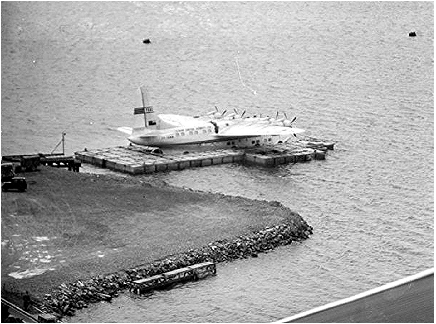
TEAL Solent Ararangi in the incomplete Evans Bay pontoon
